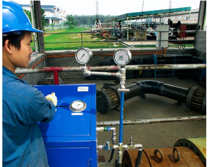
Hydrotesting of Bondstrand prefabricated pipe spool prior to shipping
