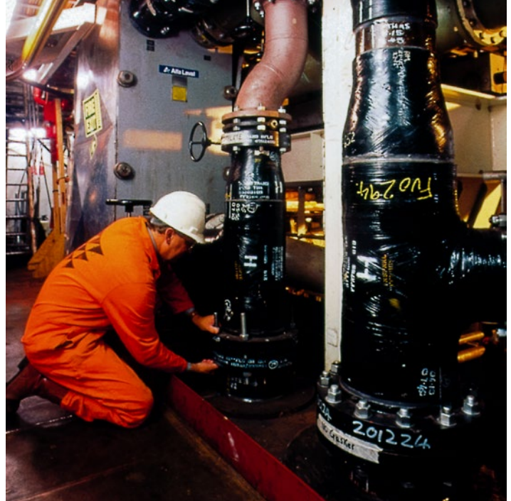
Certified installation of Bondstrand piping system
