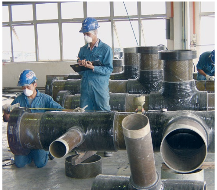
Prefabrication of custom made fiberglass spools
